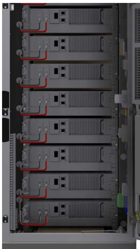
Figure 4.27 Battery cables
