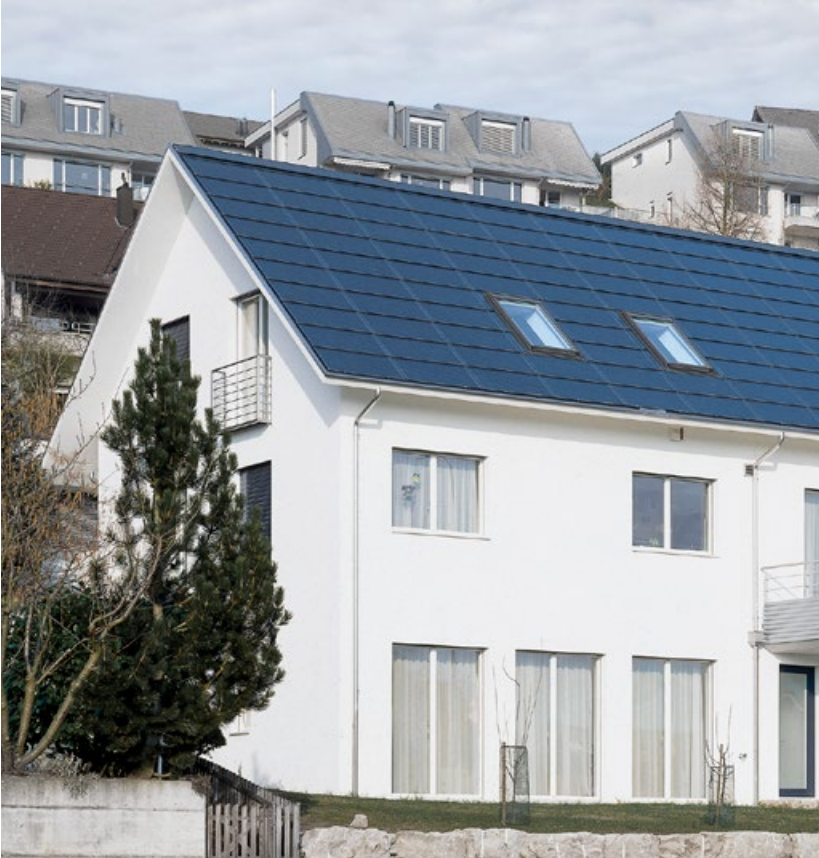
Single-family home Obersiggenthal (Switzerland)
