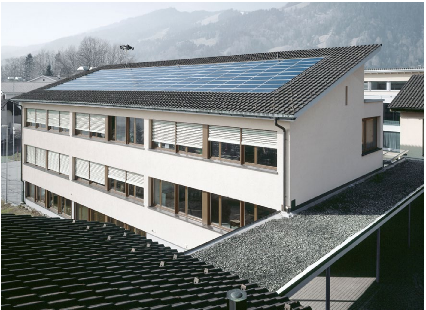
Eggeli school building Sattel (Switzerland)
